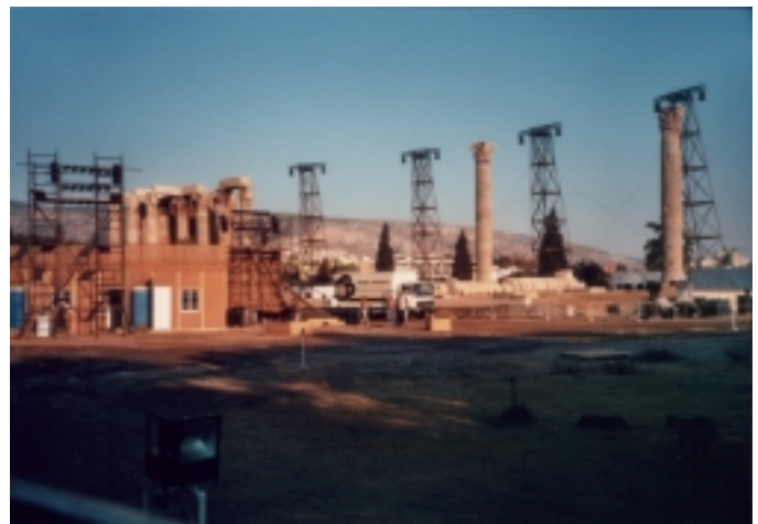
FIG. 3. Scaffolding and steel towers to support the large screen for images projection ( www.vangelis.myweb.nl/mythodeagallery.htm ).
