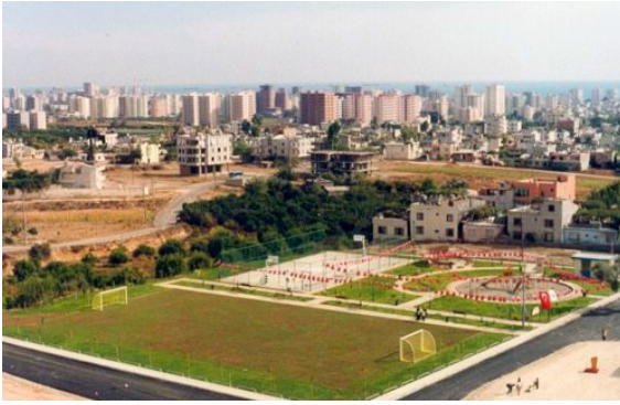
Figure 2. A scene of the high rise buildings under construction in Yenisehir town
